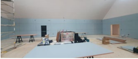
Work on the interior of the centre.
