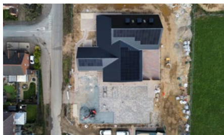
Aerial view of the exterior progress.
